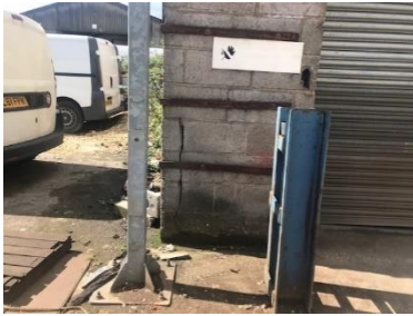
Cracking and retaining bars
