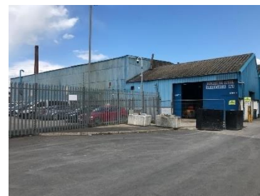
Unit 1 – front access
