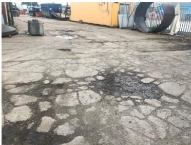
Cracking and retaining bars
