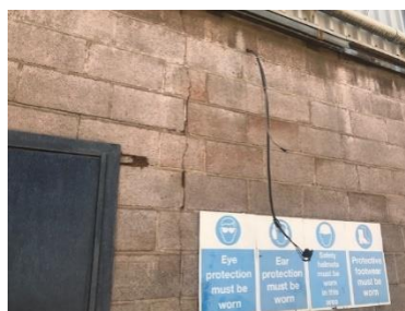
Cracking
