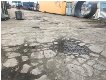
Cracking and retaining bars
