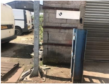
Cracking and retaining bars
