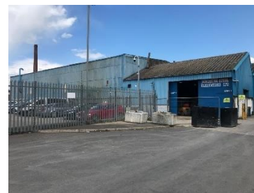
Unit 1 – front access
