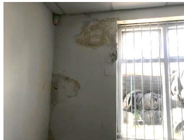
Water ingress in offices causing plaster damage
