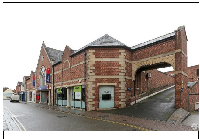
Elevation from Guildhall Street
