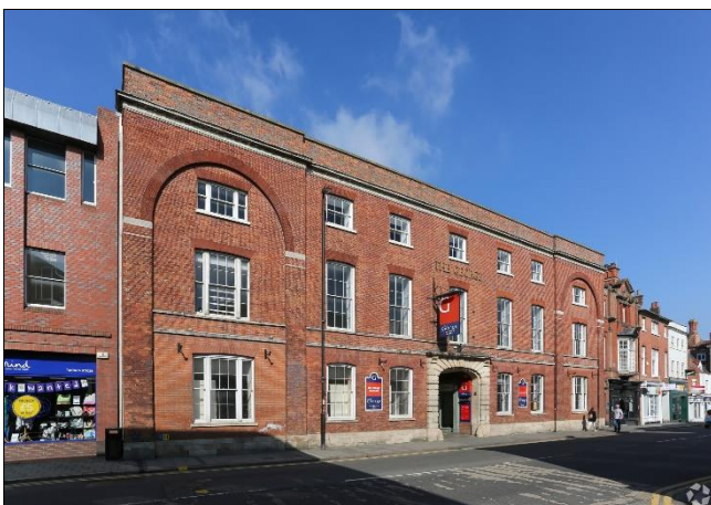
Original George Hotel Elevation from High Street
