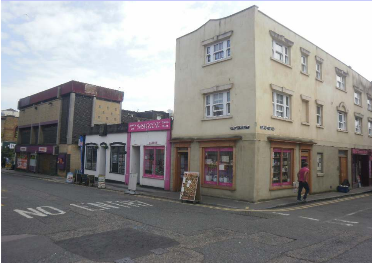
The 4 Broad Street & 7 Turner Street Building As A Whole
